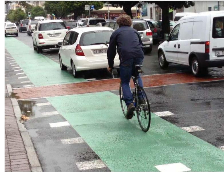
StreetBond CL skid resistance and visibility in rainy conditions along Bree Street, Cape Town.
