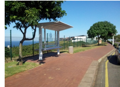
Bus Shelter next to Sidewalk
