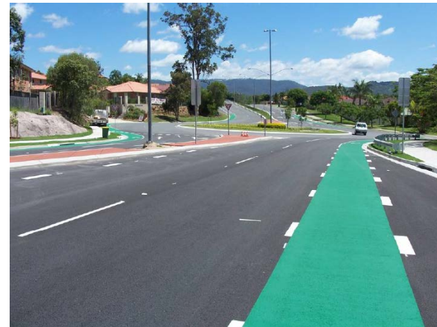
On-grade StreetBond CL Cycle Lane Application in Brisbane, Australia
