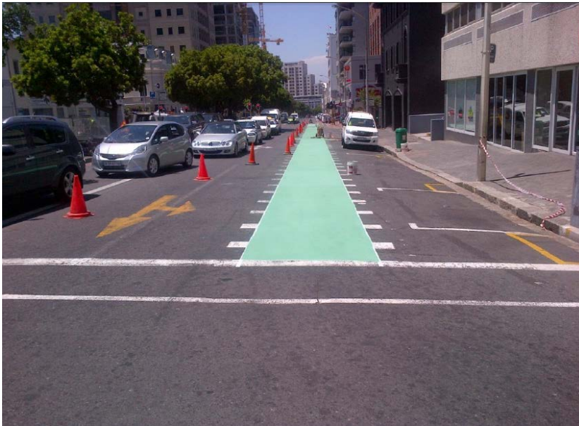
StreetBond CL Cycle Lane Application along Bree Street, Cape Town.
